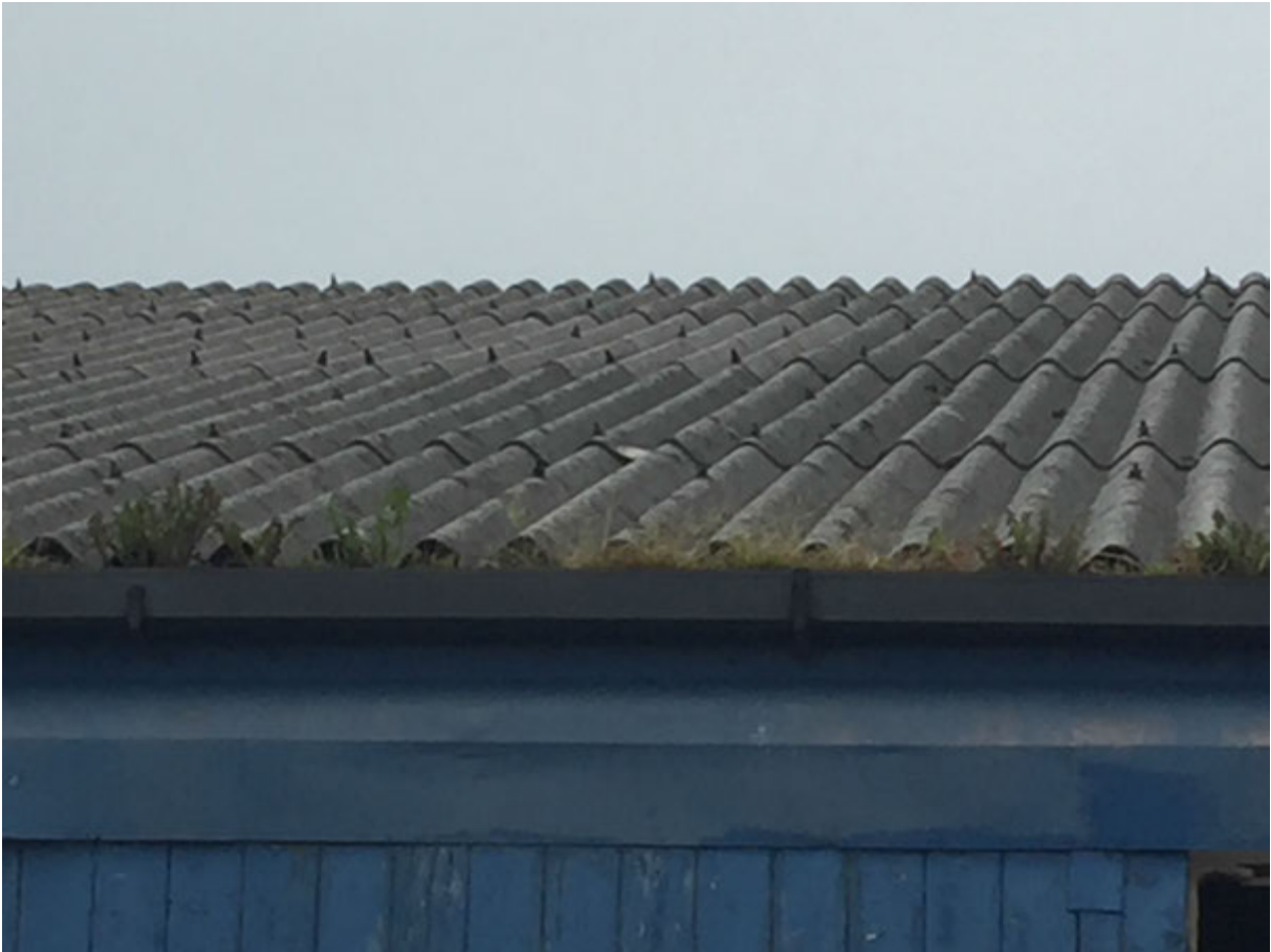
1. Position and condition of external sheets
